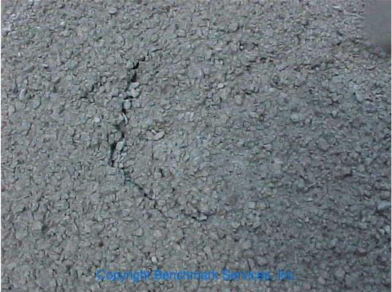
**Figure 3 - Hail Damaged granule surfaced SPUR Roof**
